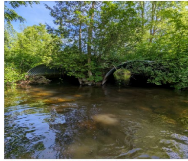
Photo 2 - View of South Culvert Ends.
