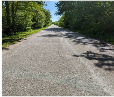
Photo 1 - View of Structure Facing East.
