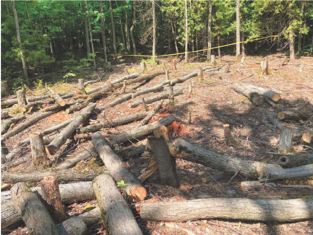
Photo No. 3: Tree clearing area looking west from County Rd, May 2024
