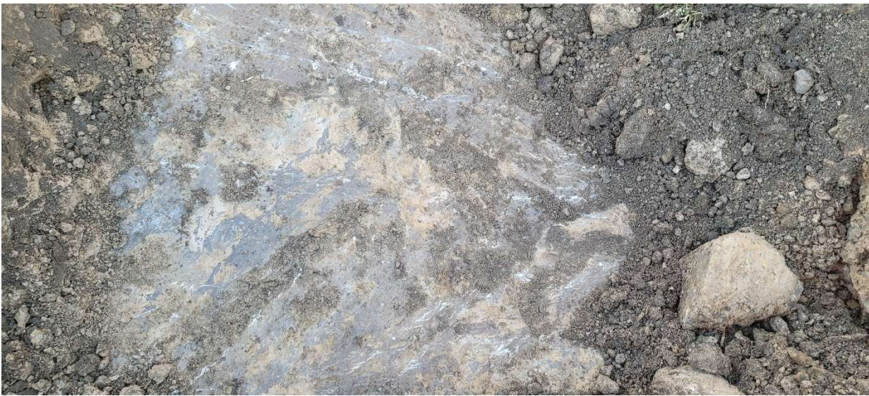
Picture 2: TH-01 – Close up view of bedrock surface.
