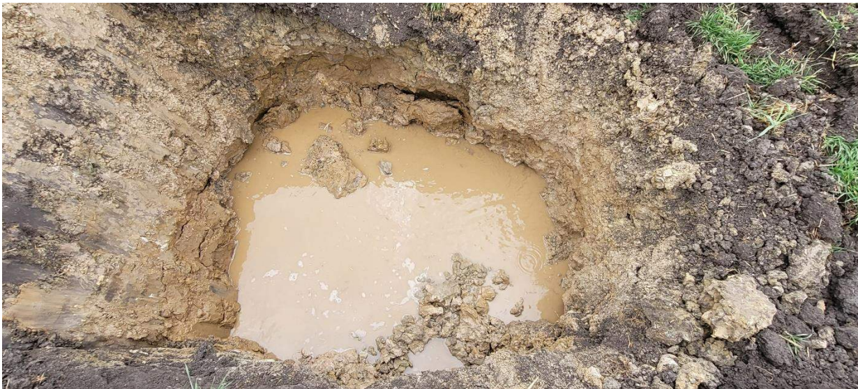
Picture 4: TH-02 – Close up view of testhole bottom.
