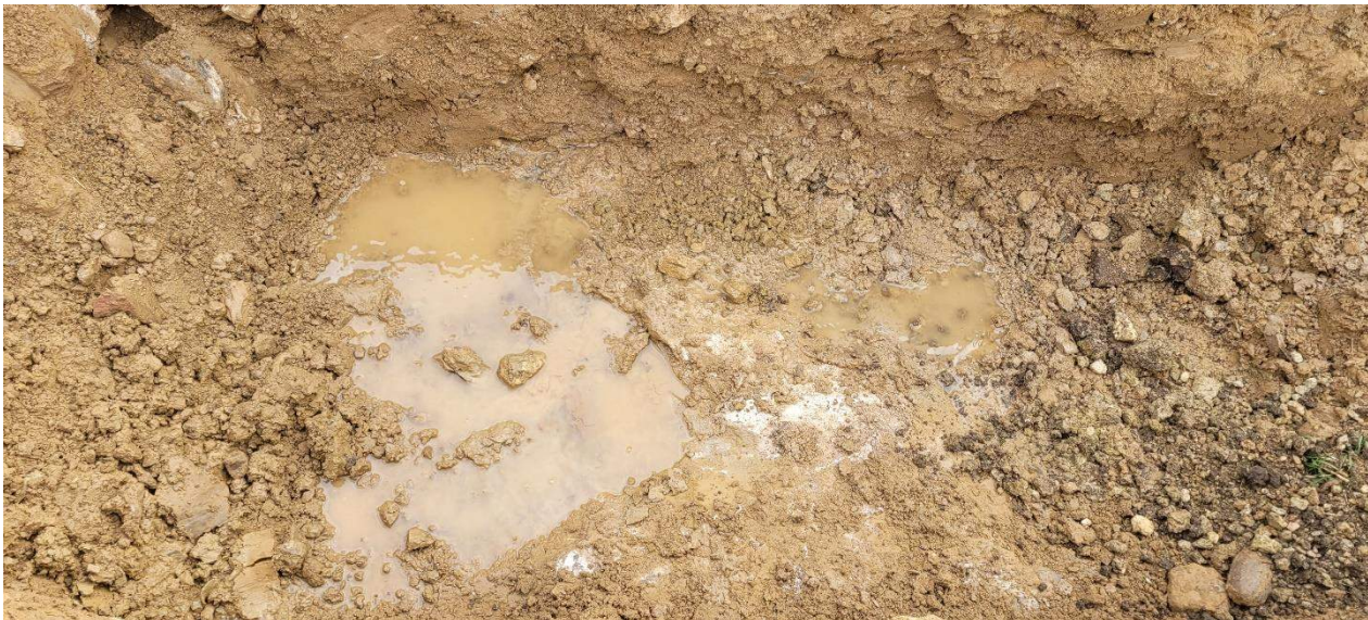
Picture 17: TH-06 - Close up view of testhole bottom.
