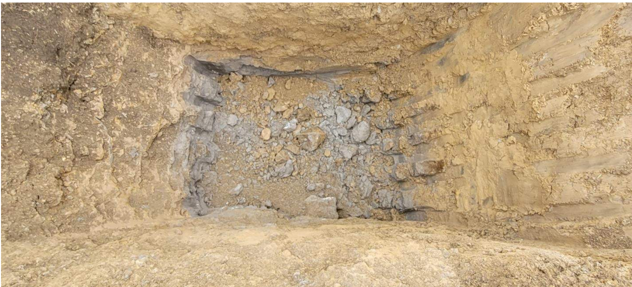
Picture 8: TH-03 - Close up view of testhole bottom.
