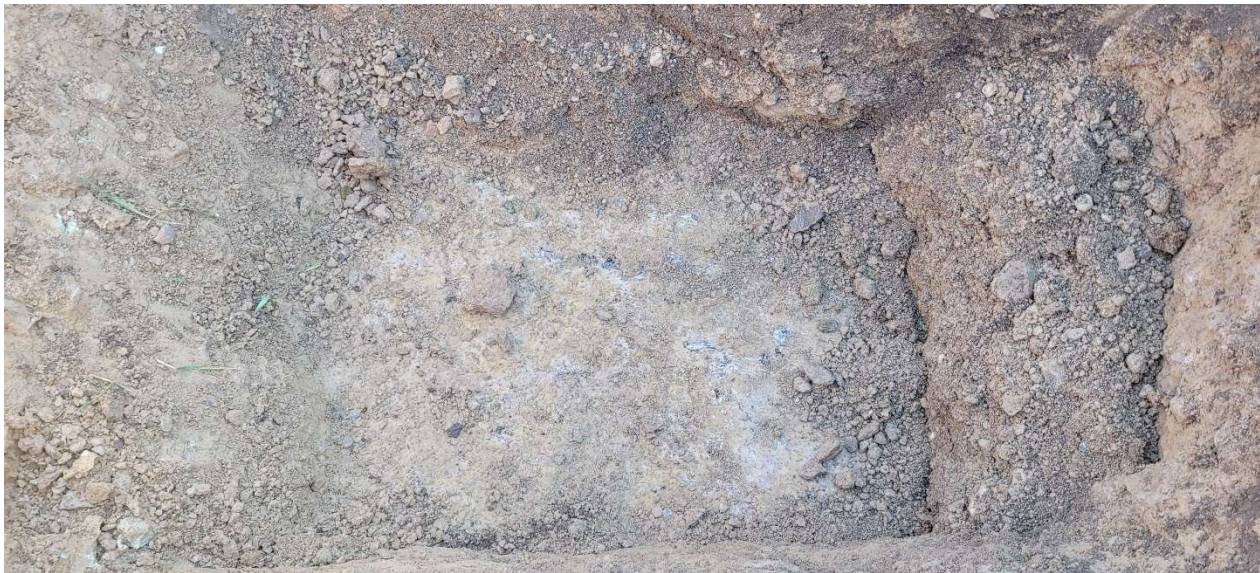
Picture 11: TH-05 - Close up view of bedrock surface.
