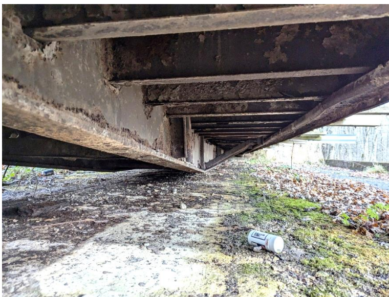
Figure 5.1: Eastern Steel Plate Girder
