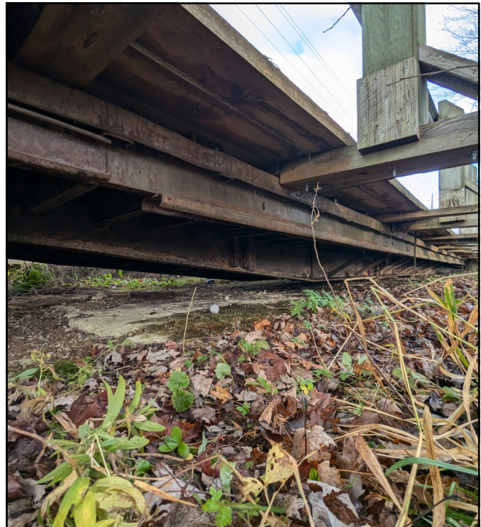
Photo 8 - View of Underside of Deck Cantilevered Edge and Steel Frame.
