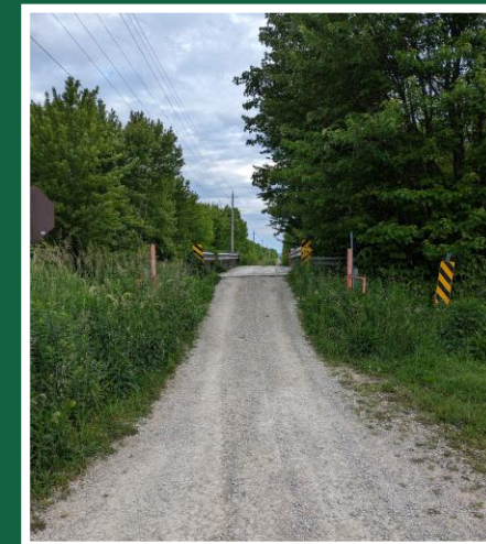
View of Approach Facing North
