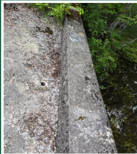
View of Concrete Curb and Deck Top
