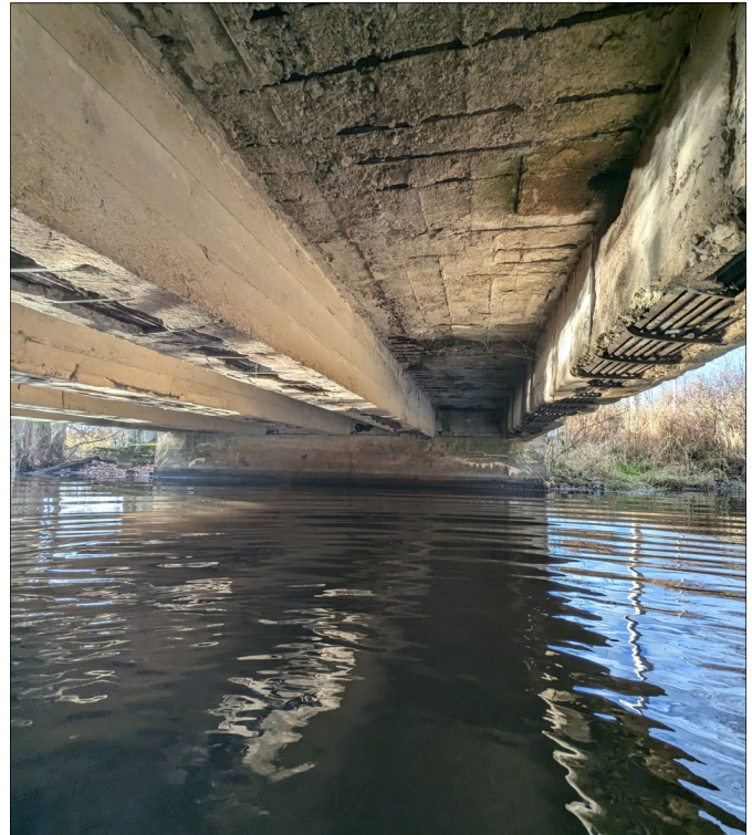
Photo 6 - View of Concrete Structure Interior Soffit.
