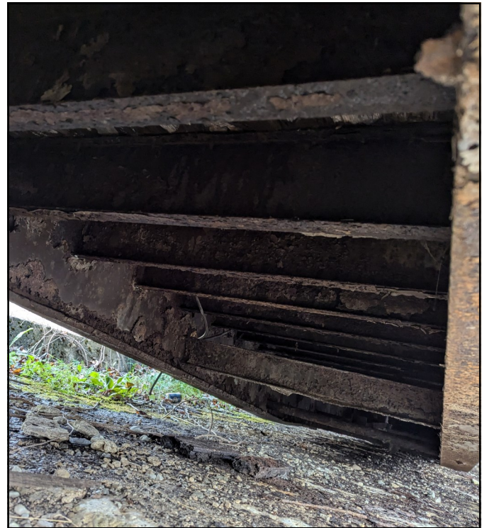
Photo 12 - View of Interior Floor Beams.
