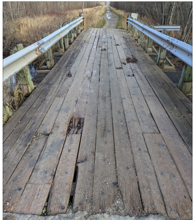
Photo 4 - View of Structure Facing North.
