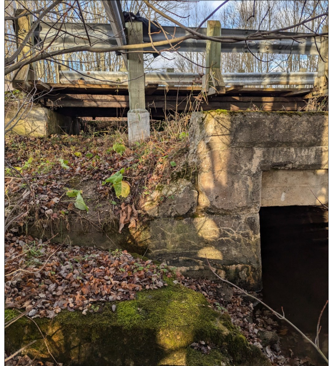
Photo 14 - View of Southeast Wingwall of Original Structure.
