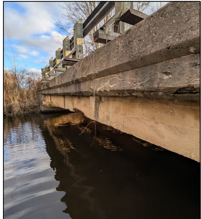
Photo 16 - View of Fascia and Curb of Original Structure.
