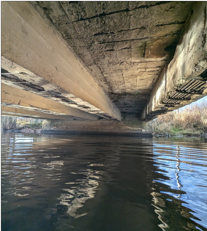
Photo 15 - View of Interior Soffit of Original Structure.
