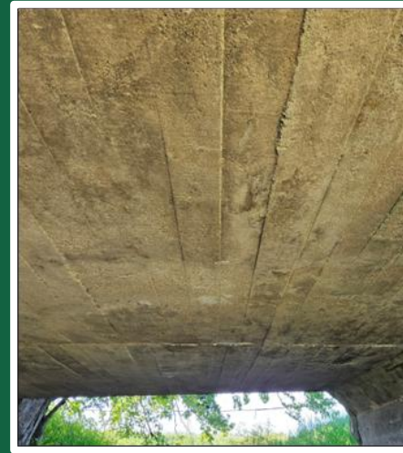
View of Interior Soffit
