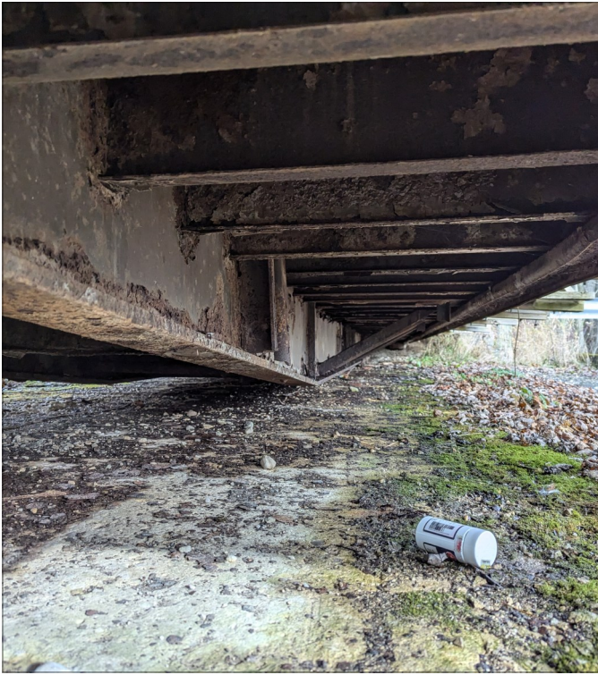
Photo 9 - View of Cantilevered Floor Beams.
