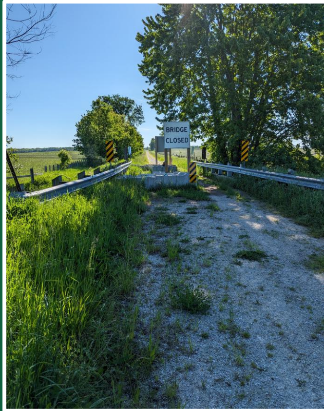
View of Structure Facing East
