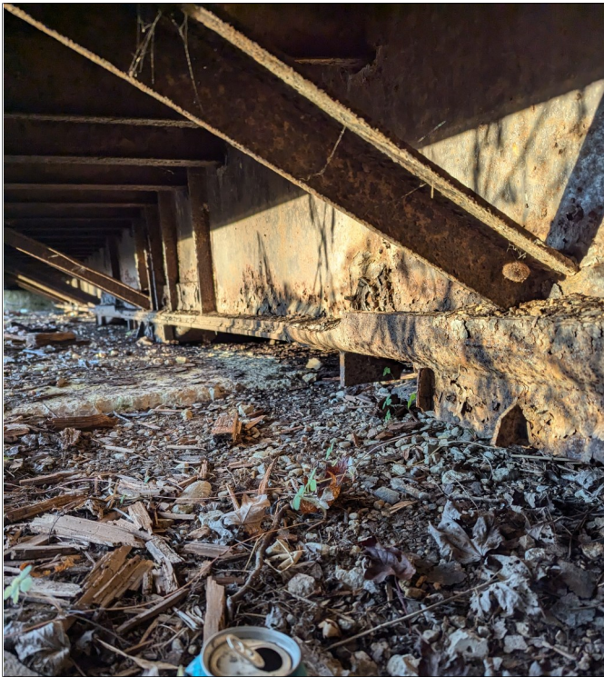
Photo 11 - View of Steel Girder and Diagonal Strutting.
