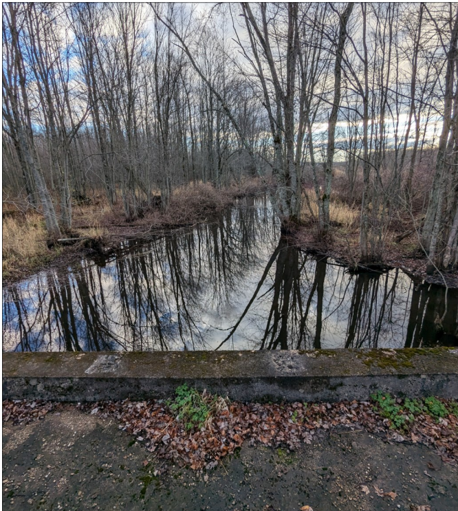
Photo 7 - View of Waterway Facing East.
