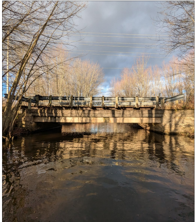
Photo 2 - View of Structure Facing West.
