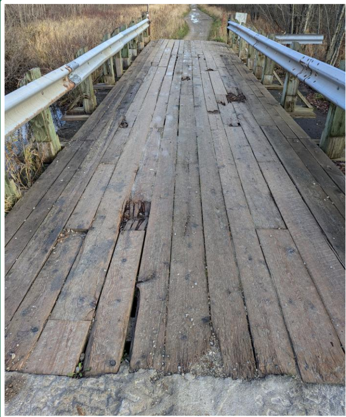
View of Structure Facing North
