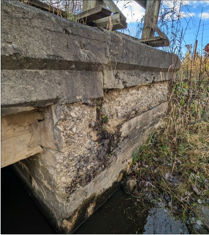
Photo 13 - View of Southwest Wingwall of Original Structure.
