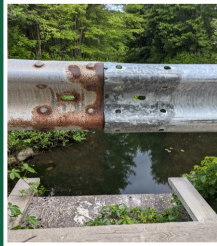
View of Barrier Lap Splice
